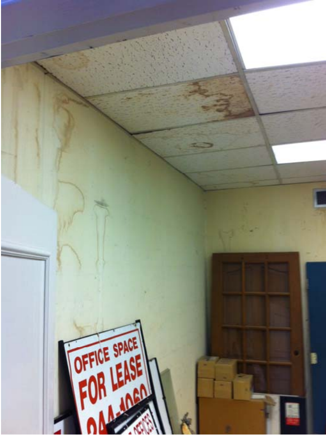
Picture # 7 – Interior Water damage above studio
