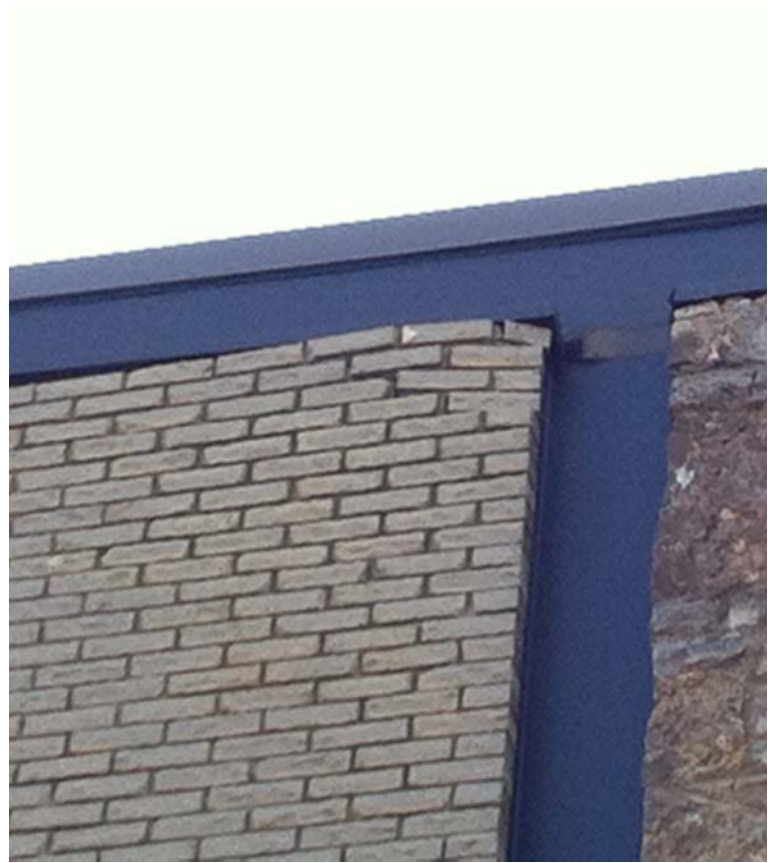
Picture #8 – Exterior Brick Veneer Failure
